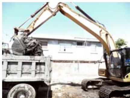
A backhoe clearing the land.
