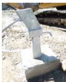
The new well at the construction site.
